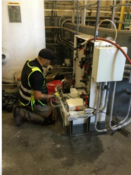
Retrofit of Existing Ferric Sulfate Chemical Feed Skid with new pumps
