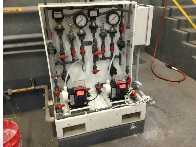
Retrofit of Existing Ferric Sulfate Chemical Feed Skid with new pumps
