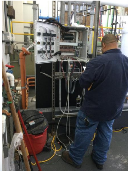
New Sodium Bisulfite Skid Installation and testing
