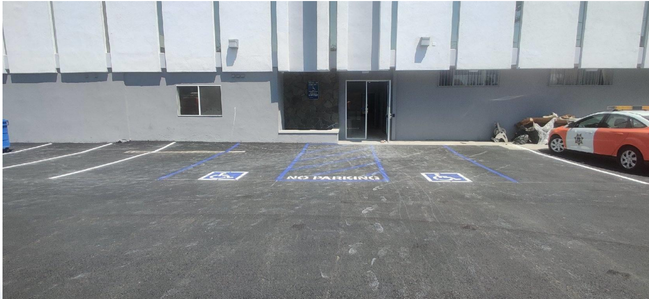
Parking Lot Striping
